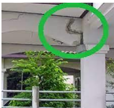
Fig.1.3. Shrinkage crack
