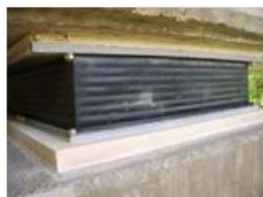
Fig. Elastomeric bearing
