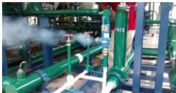
Fig. 2.1 Cryogenic PRV in operation at LSSF
