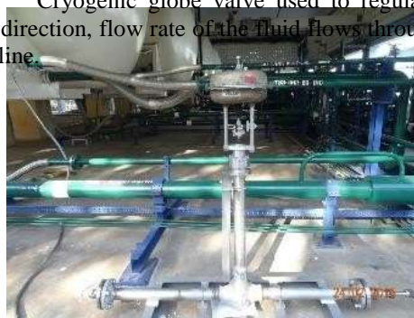
Fig. 4.3 Cryogenic globe valve
