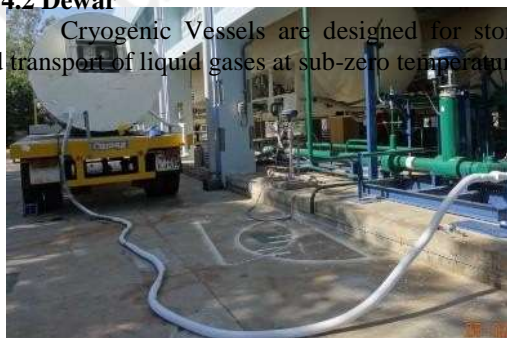
Fig. 4.2 Liquid nitrogen storage tank at operation
