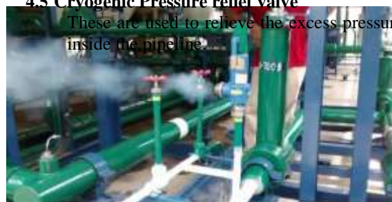
Fig. 4.5 Cryogenic pressure relief valve
